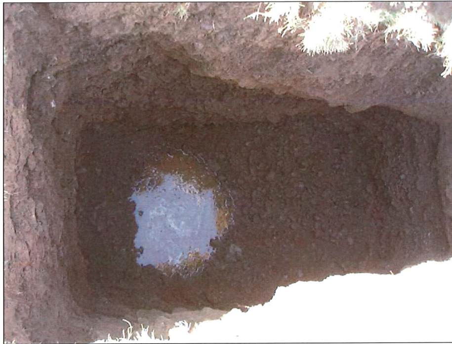
Photo 3: Ground Water Seepage in Test Pit TP5
