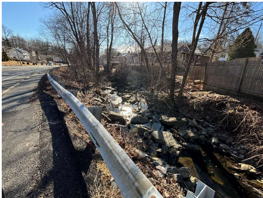
Photo 5. Downstream (easterly) view of D-Series stream flowing parallel to Pleasant Street.
