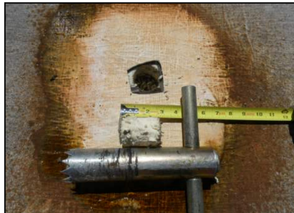
Photo Core #2 - DHCI—Dining Roof Area 2
