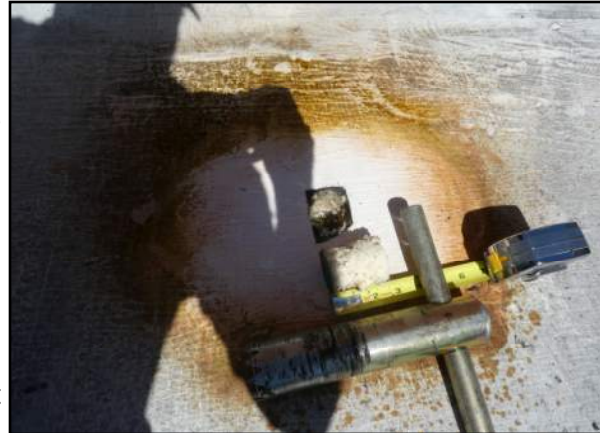
Photo Core #1 - DHCI—Dining Roof Area 2
