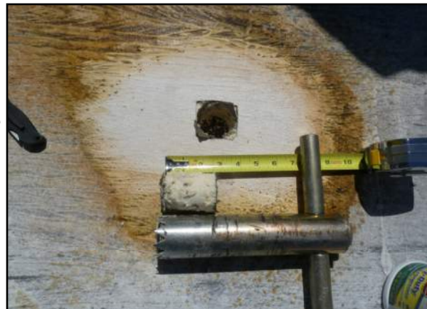
Photo Core #2 - DHCI—Dining Roof Area 3
