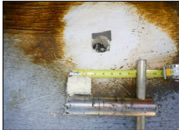
Photo Core #1 - DHCI—Dining Roof Area 3
