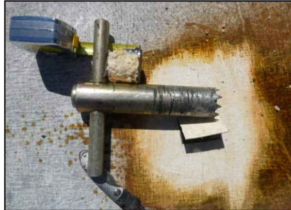
Photo Core #1 - DHCI—Dining Roof Area 1
