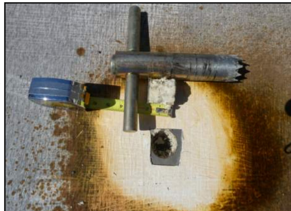
Photo Core #2 - DHCI—Dining Roof Area 1
