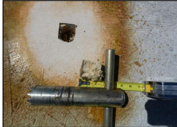
Photo Core 1 - DHCI—Dietary Roof Area 4
