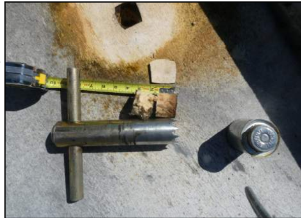
Photo Core 1 - DHCI—Dietary Roof Area 11
