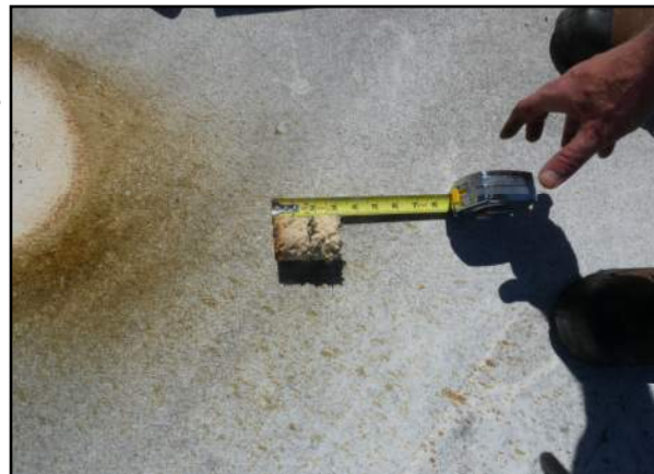
Photo Core 2 - DHCI—Dietary Roof Area 10
