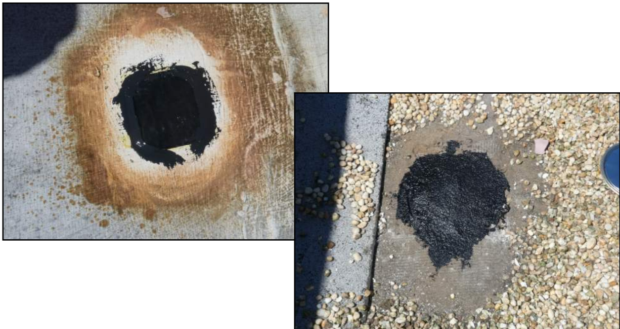
Photos 1 - 2 - Typical roof core repairs
