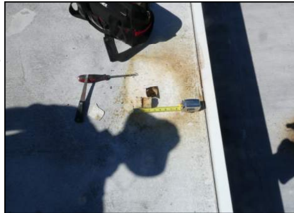
Photo Core 1 - DHCI—Dietary Roof Area 10
