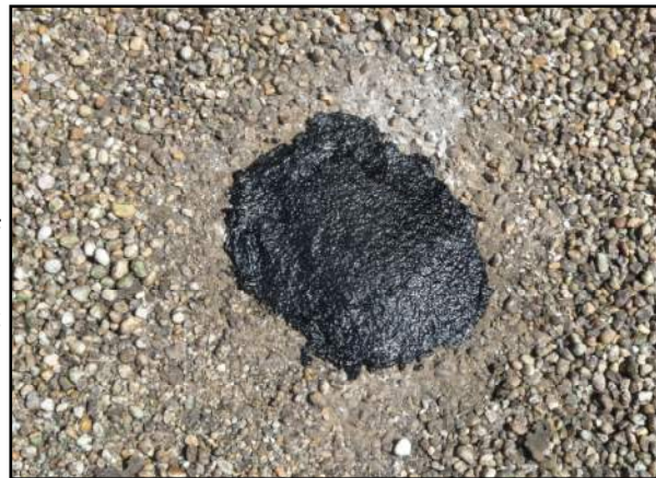
Photo Core 2 - DHCI—Dietary Roof Area 8
