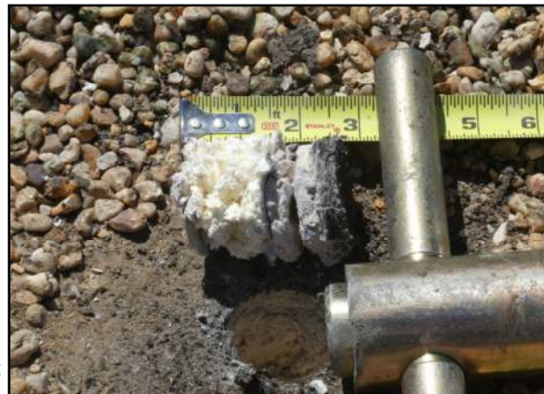
Photo Core 2 - DHCI—Dietary Roof Area 6
