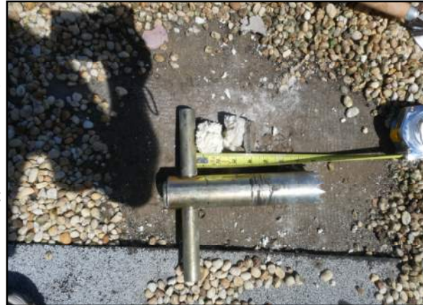
Photo Core 1 - DHCI—Dietary Roof Area 6
