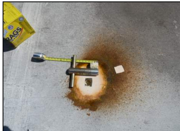
Photo Core 2 - DHCI—Dietary Roof Area 9
