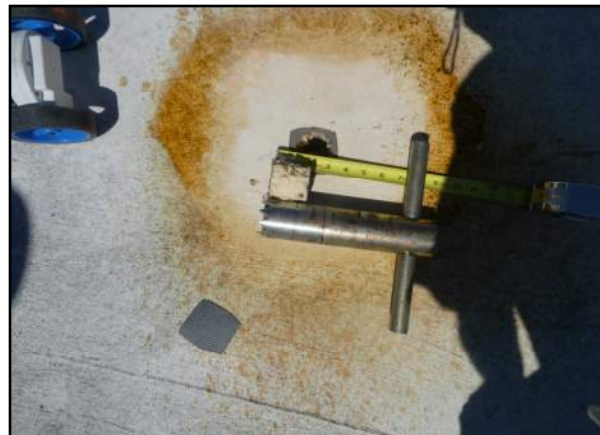
Photo Core 2 - DHCI—Dietary Roof Area 4
