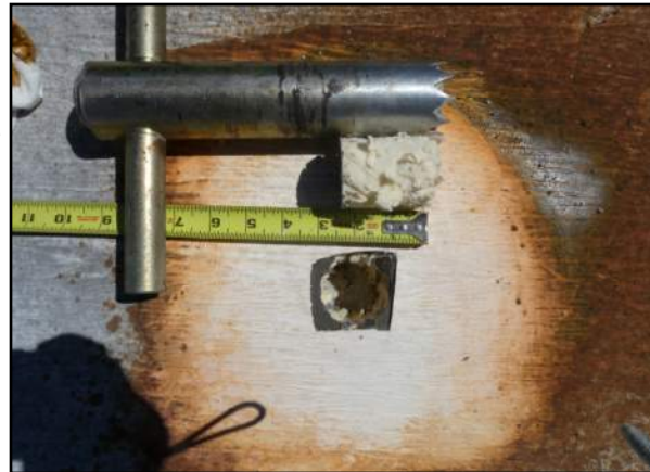
Photo Core 1 - DHCI—Dietary Roof Area 9
