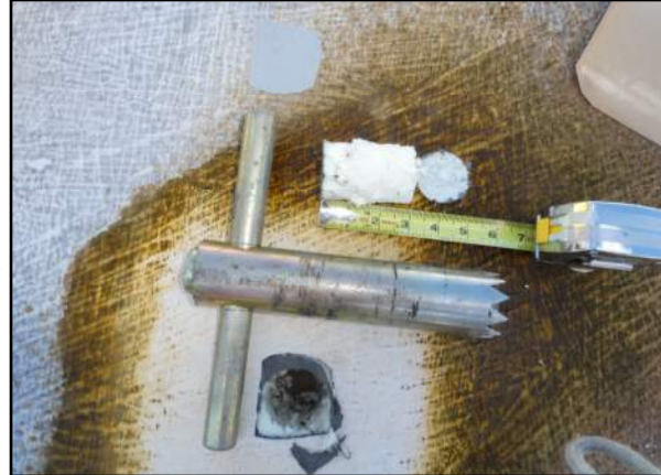
Photo Core 2 - DHCI—Dietary Roof Area 5
