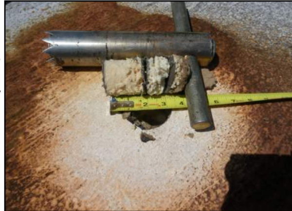
Photo Core 1 - DHCI—Dietary Roof Area 5
