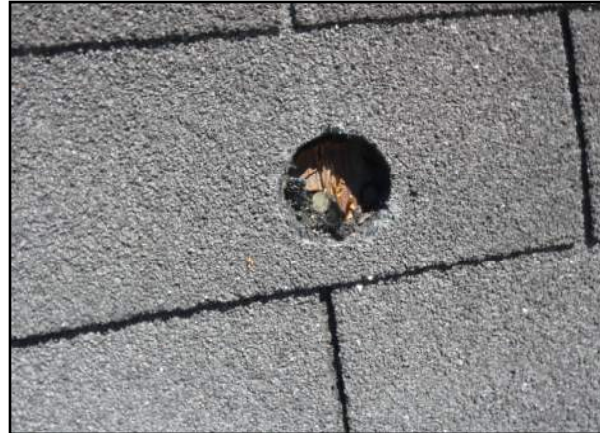
Photo Core 1 - DHCI—Dietary Roof Area 7
