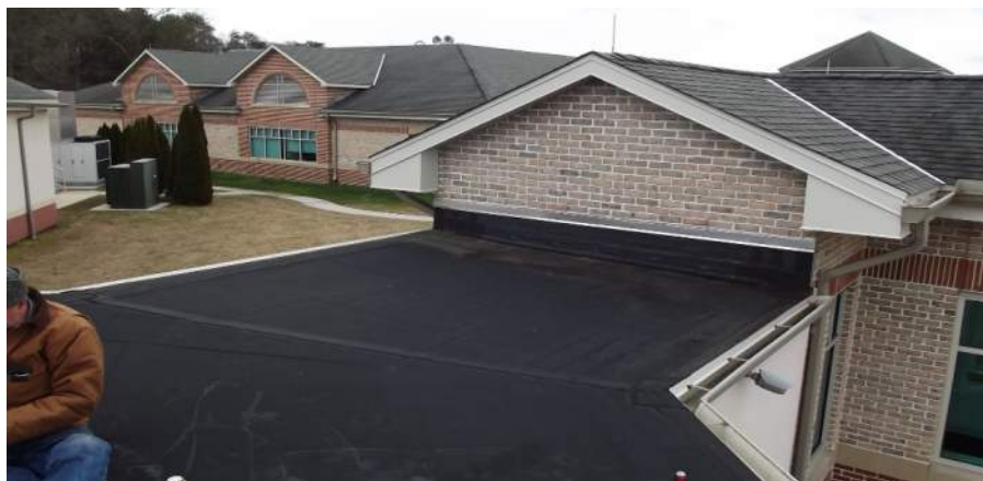
Photo 23 – Therapy Pool Corridor Roof Overview
