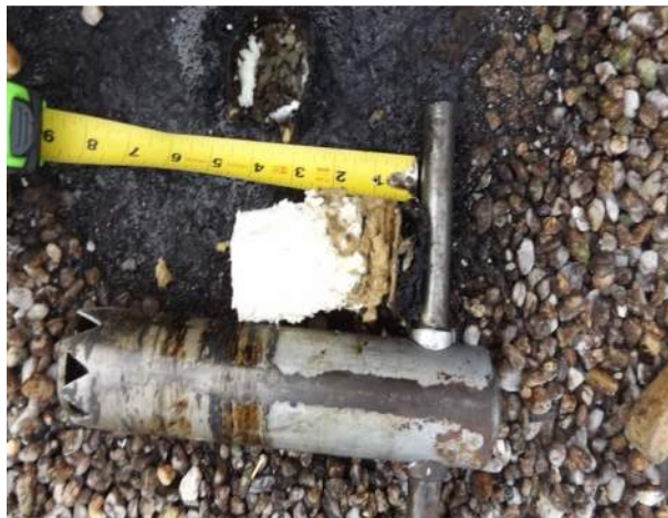
Roof Core Admin. Wing RA - 1
