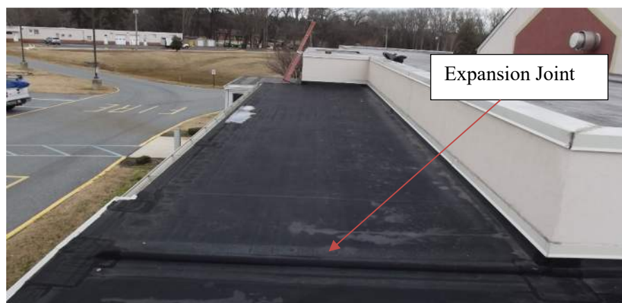
Photo 22 – Therapy Pool Corridor Roof Overview
