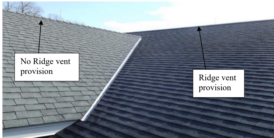
Photo 9 – Overview of shingled roof
