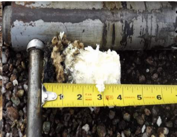
Roof Core Residential Wing RA - 11
