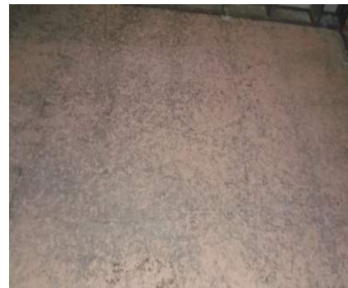
Photo 4 – Fireproofing material on floor of attic space.
