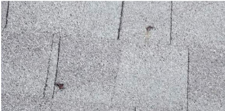
Photo 13 – Typical nail pops at shingles.
