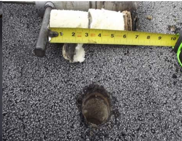
Roof Core Pool Vestibule Roof RA - 14
