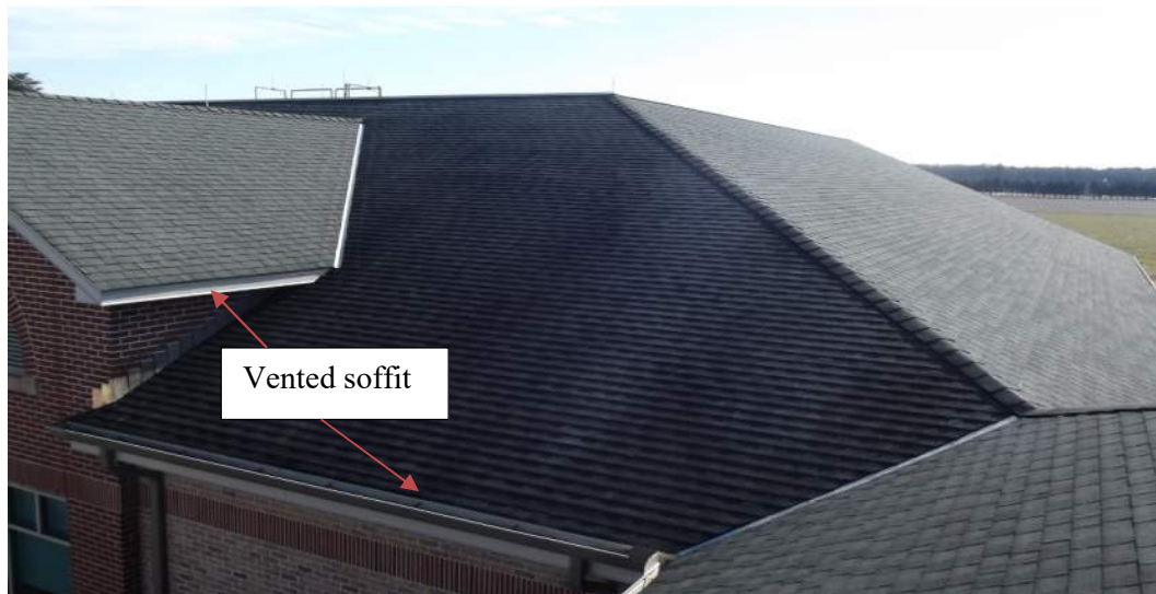
Photo 10 – Overview shingled roof
