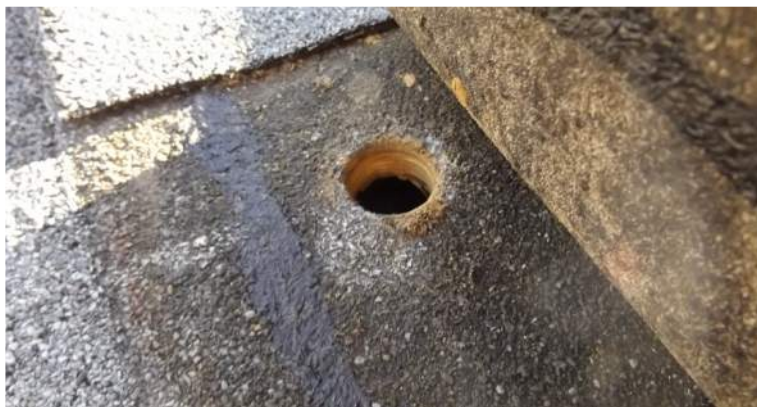
Photo 8 – Roof core taken at Therapy Pool.
