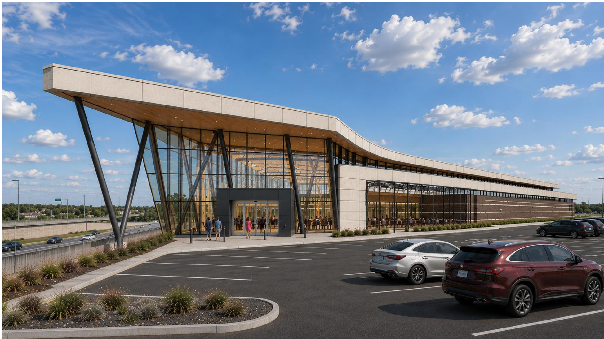
Image #1 – Exterior View
