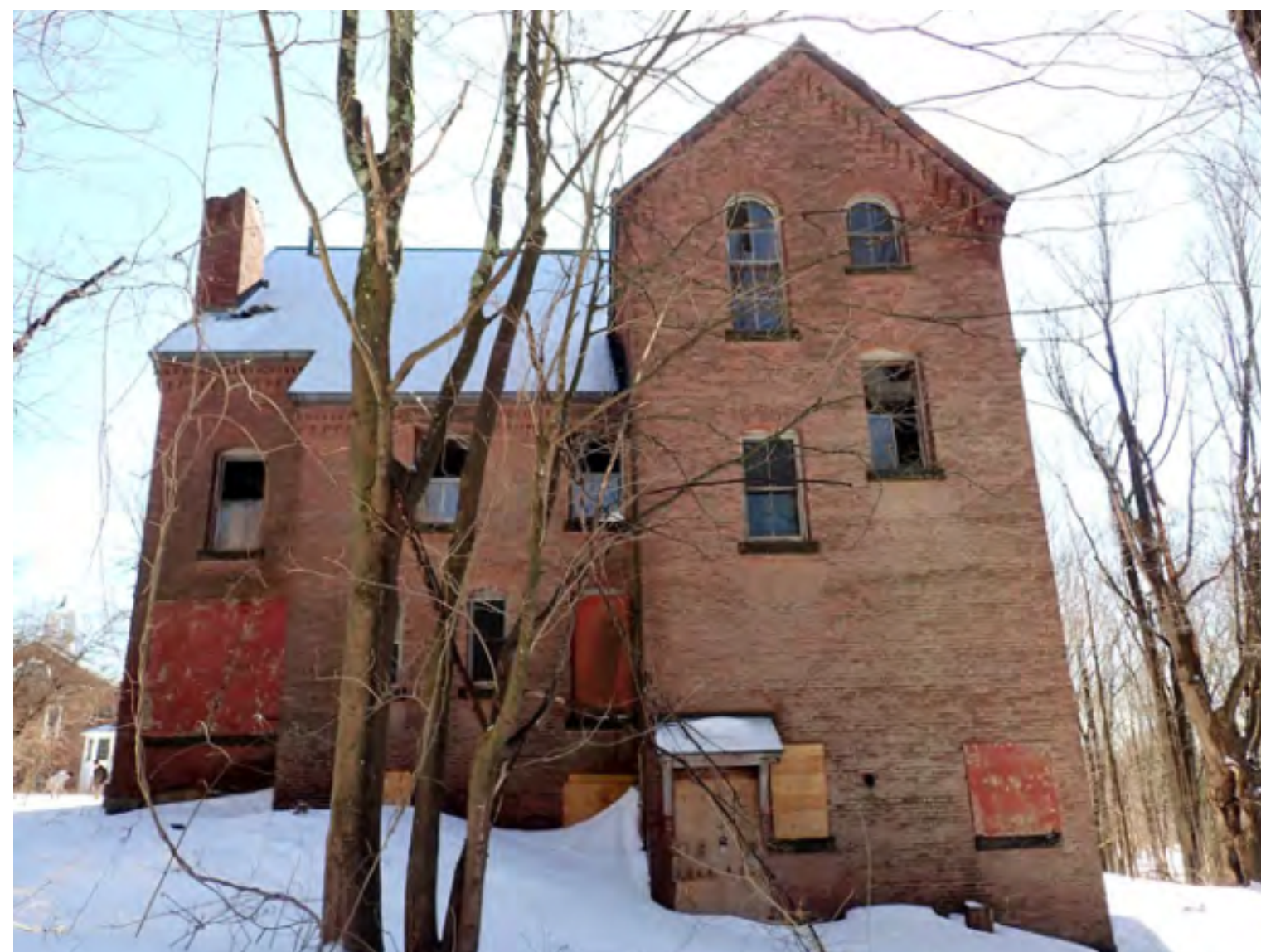
3. NORTH ELEVATION, VIEW SOUTH
