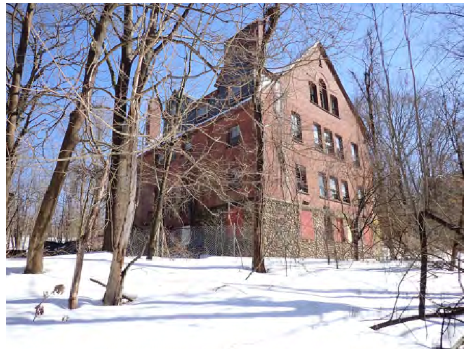
4. NORTH ELEVATION (LEFT) AND WEST ELEVATION (RIGHT), VIEW EAST
