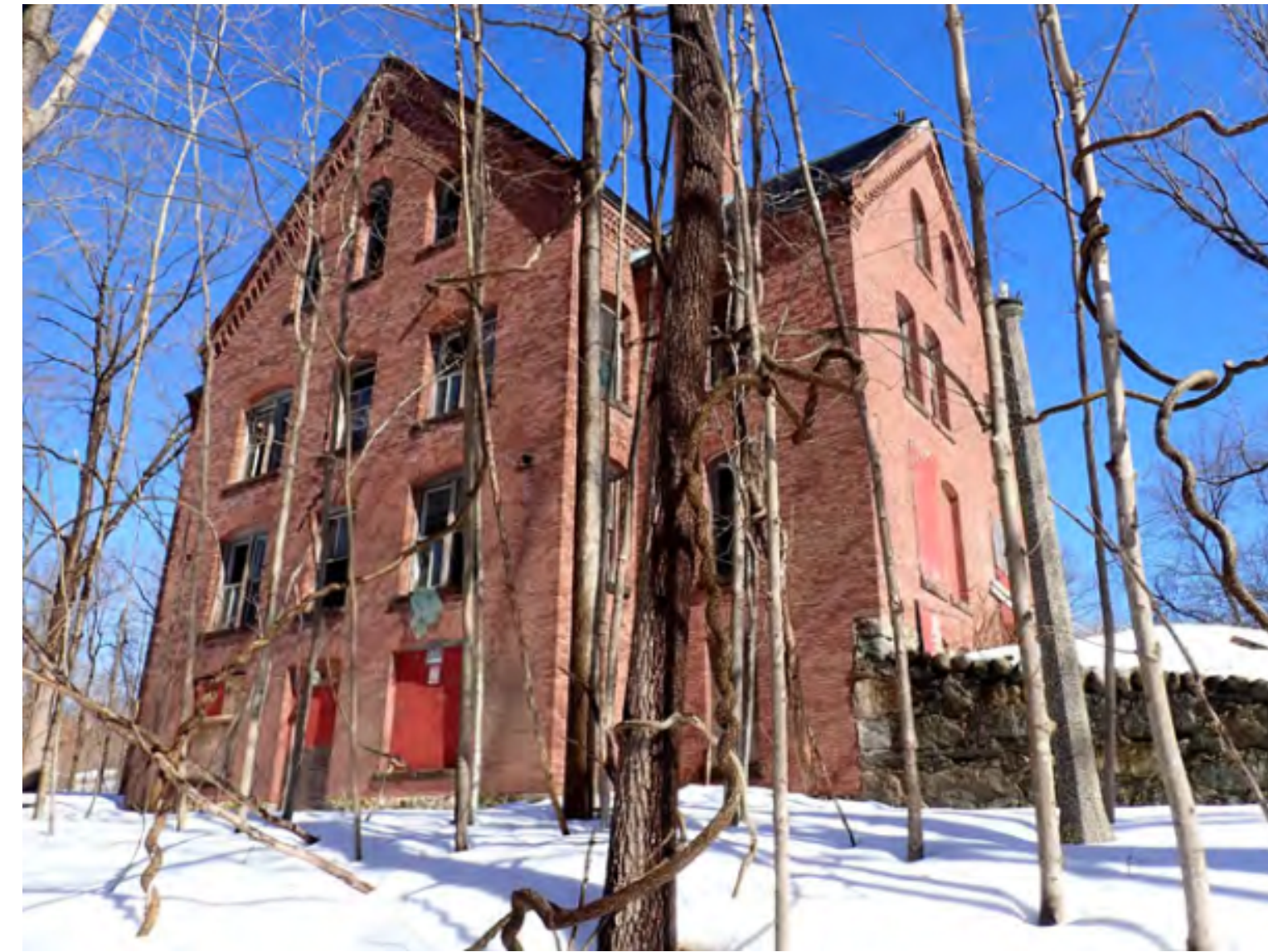
4. WEST ELEVATION (LEFT) AND SOUTH ELEVATION (RIGHT), VIEW NORTHEAST
