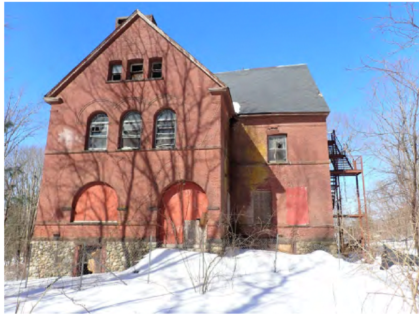
1. SOUTH ELEVATION, VIEW NORTHWEST
