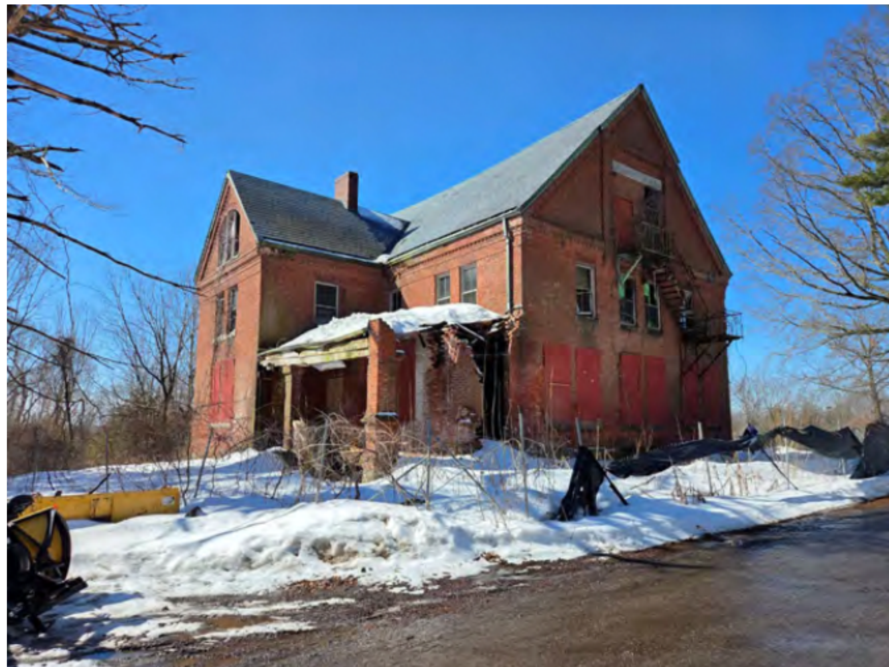
1. EAST ELEVATION (LEFT) AND NORTH ELEVATION (RIGHT), VIEW SOUTHWEST
