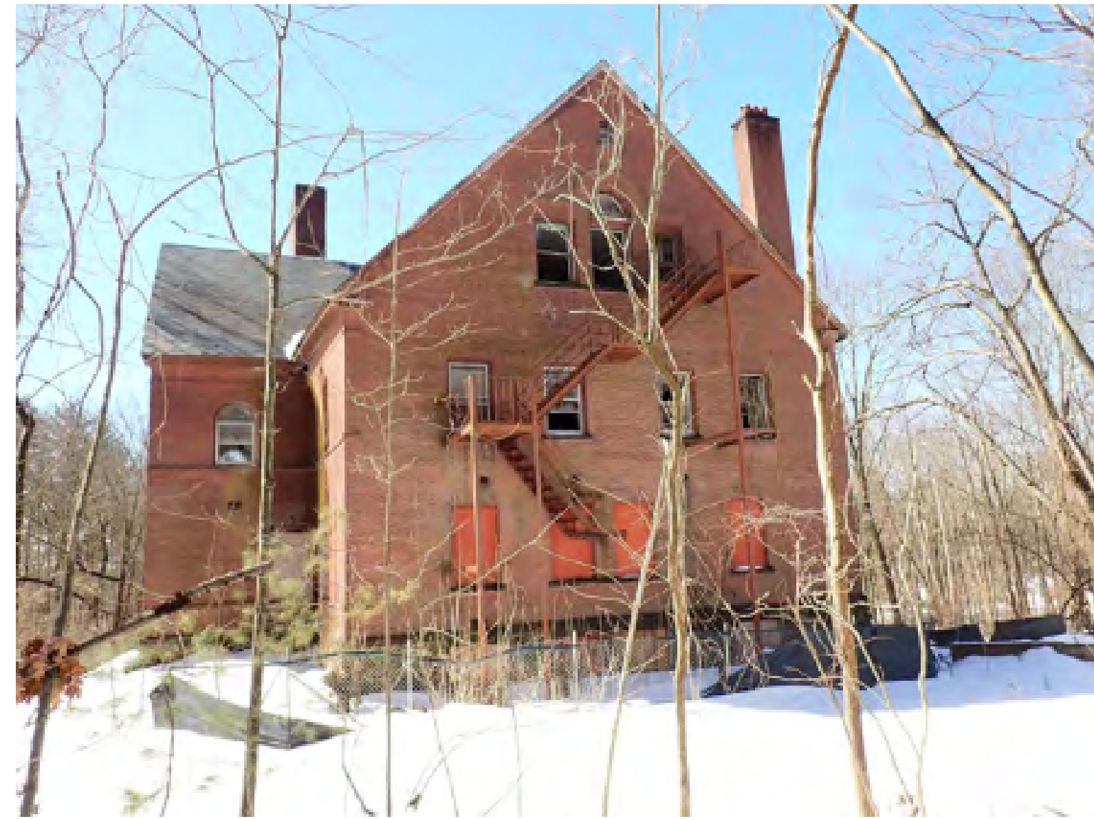
2. EAST ELEVATION, VIEW SOUTHWEST
