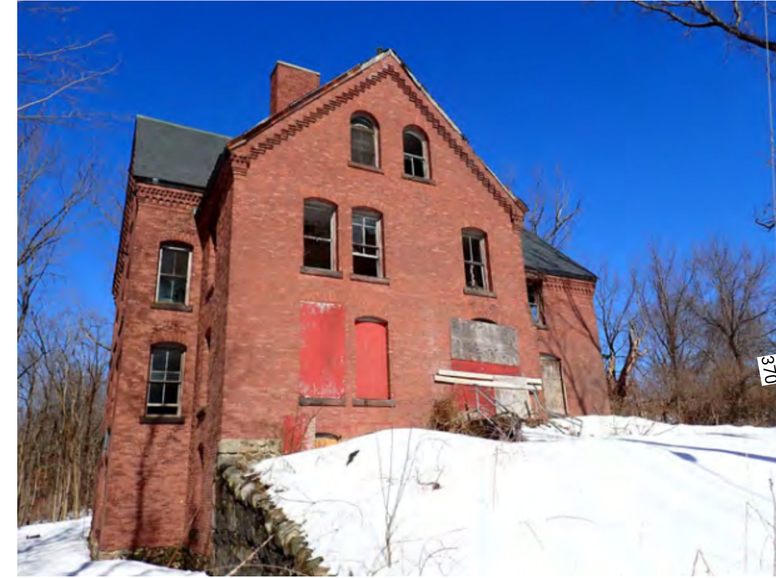
5. SOUTH ELEVATION (RIGHT), VIEW NORTH
