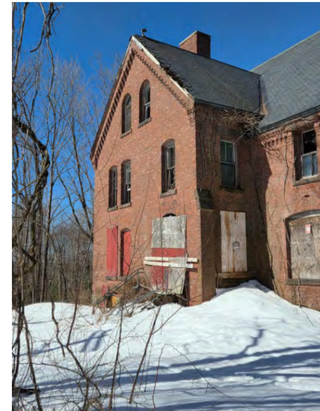
6. SOUTH ELEVATION (RIGHT), VIEW NORTHWEST
