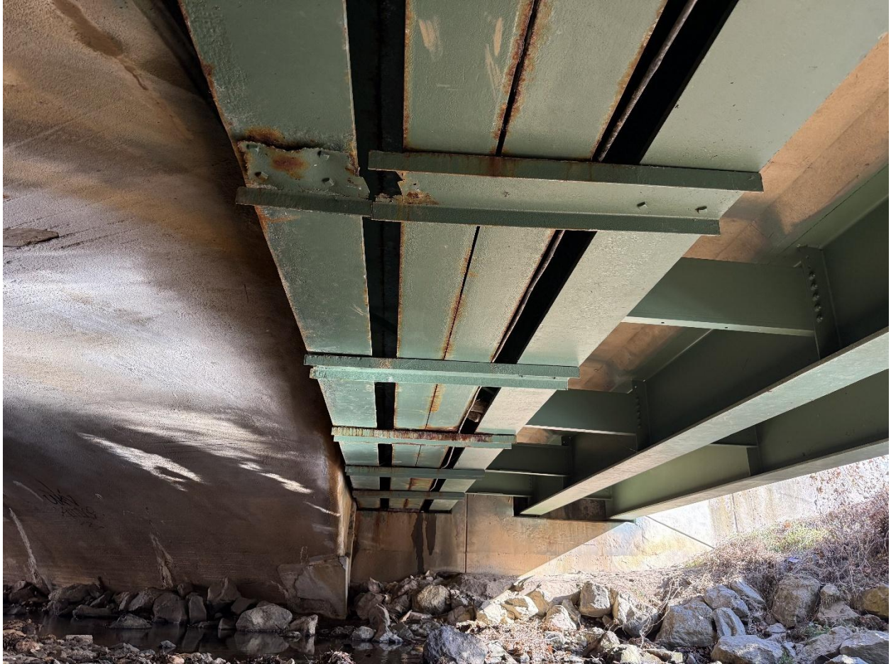
BR 1-229A (Steel channels to be removed)
