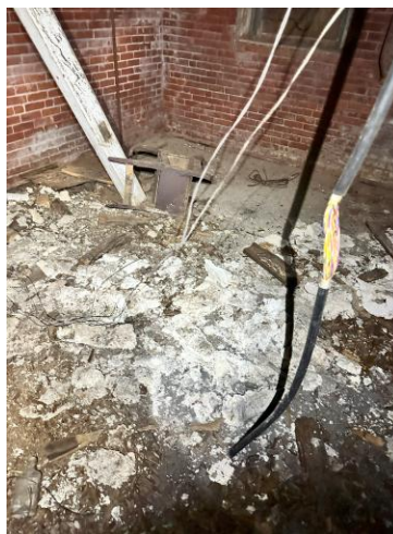
BASEMENT PIPE INSULATION DEBRIS
