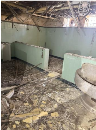
BASEMENT BATHROOM PLASTER PIPE INSULATION THROUGHOUT
