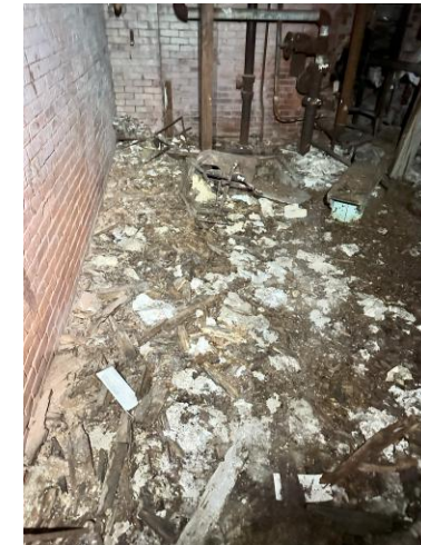
BASEMENT PIPE INSULATION DEBRIS
