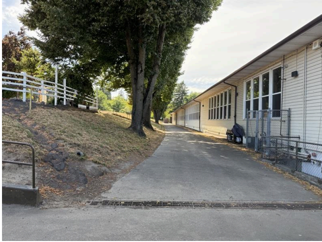
Steep slope near school entry / exit, floor drain
